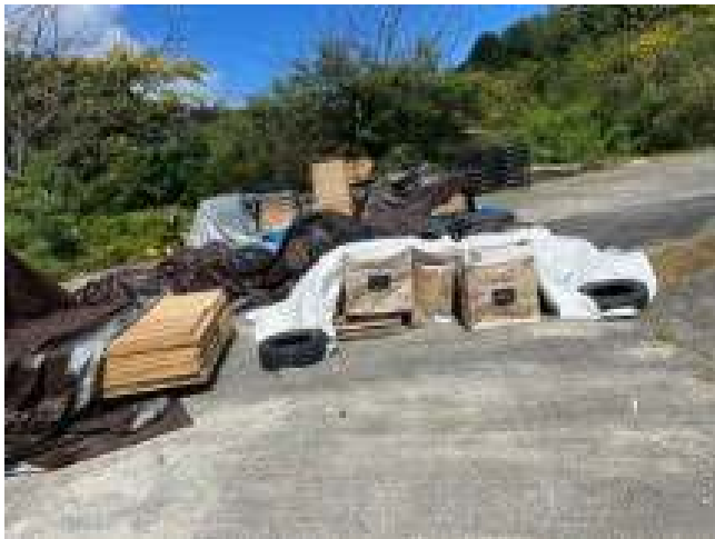
Construction material, including treated plywood, staged outside.
