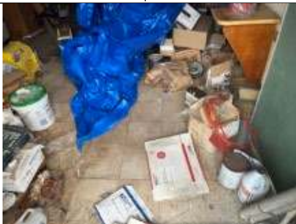
Suspected ACM material (floor tile).
