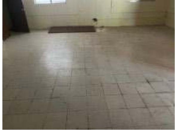
Suspected ACM material (floor tile).
