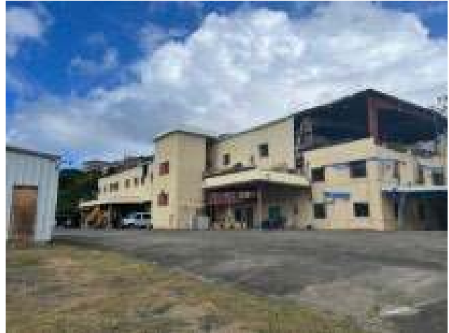
Subject Property, central office, facing Northeast.
