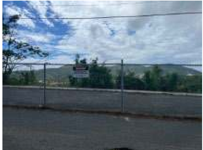
Subject Property, former Senior Center residences, facing west.
