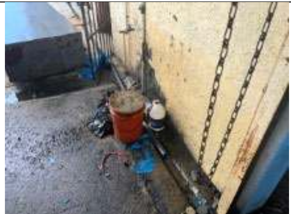
Petroleum staining around heavy equipment stored on slab.
