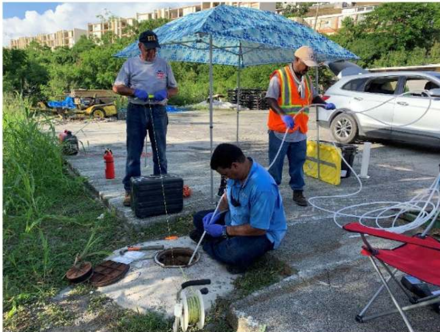
Photograph 11: EPA OSCs providing field support to START V personnel during pump setup for the sampling monitoring well MW-13D.
