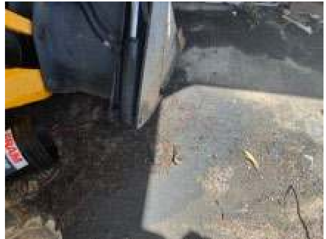
Petroleum staining around heavy equipment stored on slab.
