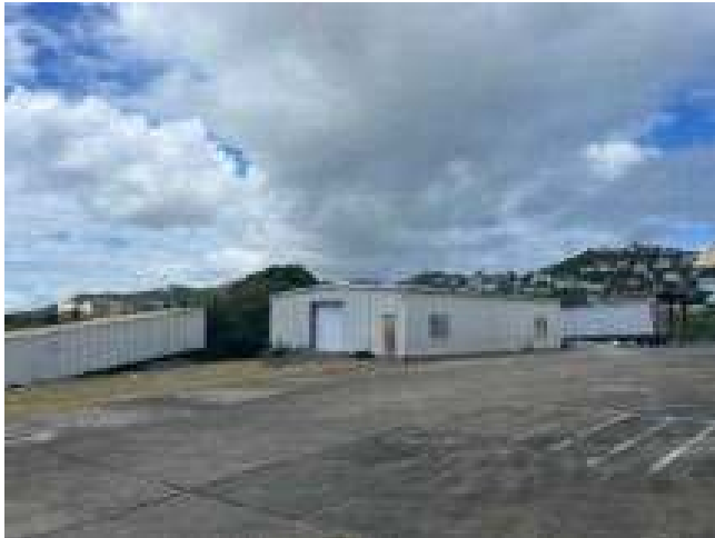
Subject Property, maintenance building, facing Northwest.
