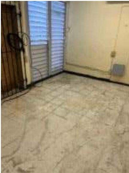
Suspected ACM material (floor tile).
